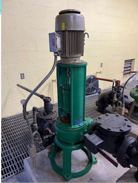
Replaced Waste Pump
