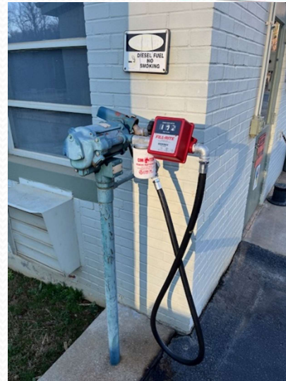
Replaced Nozzle on Diesel Pump
