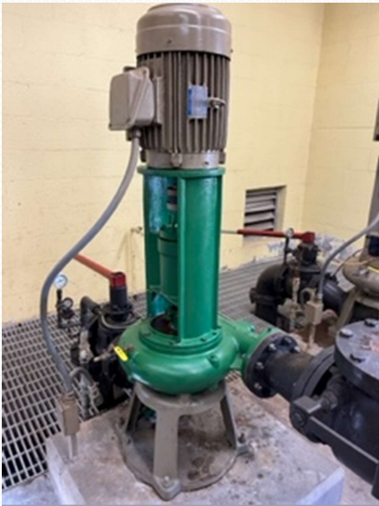
Replaced Return Pump
